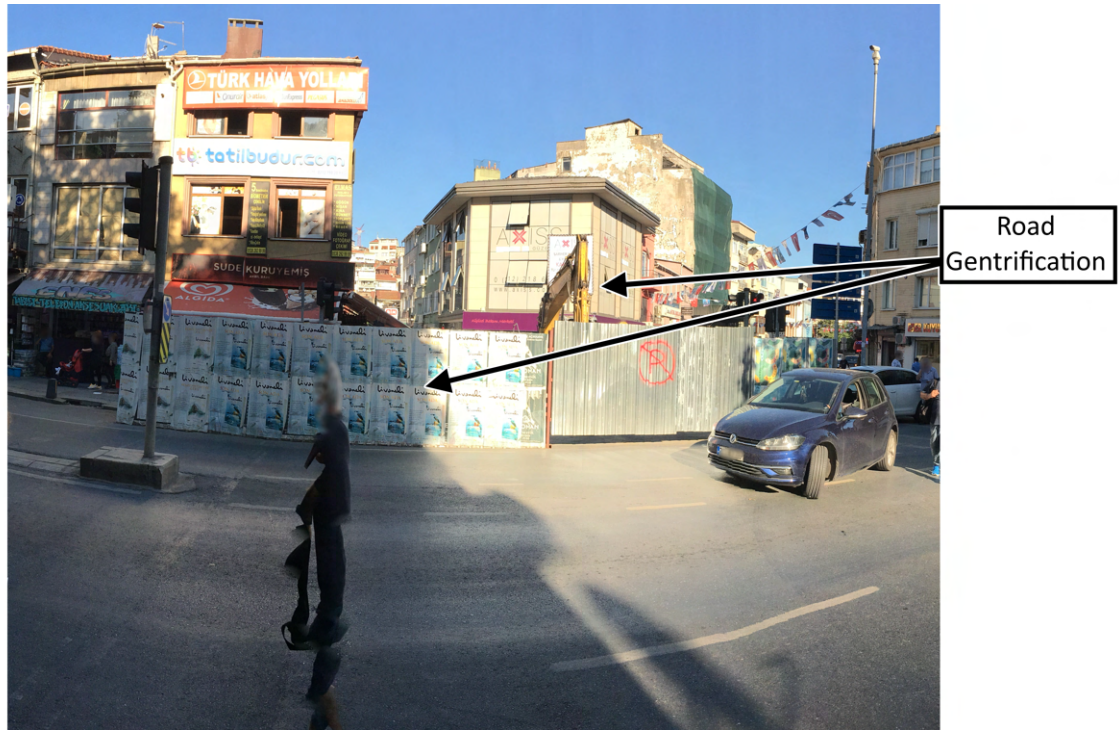
Figure 24: Road Improvement Construction in Site 9 (self-taken photograph)
