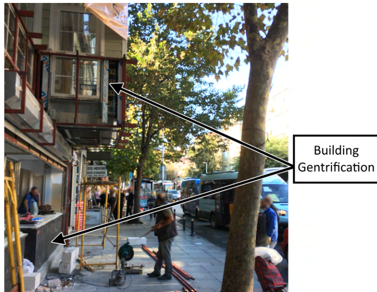
Figure 25: Building Rejuvenation in Site 10 (self-taken photograph)
